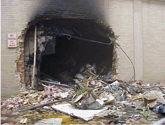
Fig. 13-3. Earliest known photo, by a DoD photographer, of the near-perfectly-round 9- to 12-foot diameter alleged “exit” hole in the inner wall of the middle C Ring.
