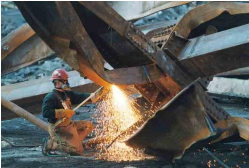
Above – a worker at ground zero cuts one of the remaining steel columns in order to facilitate its removal.
